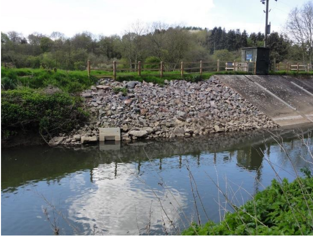
Eel Pass upstream of Flume
